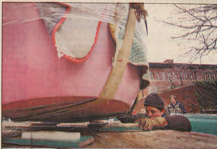
Todd Bowman of the Frank Lucco Co. positions supports under the Q before it is hauled away while the Akron Art Museum is expanded.
